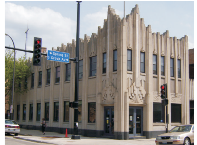
Image of existing building.
