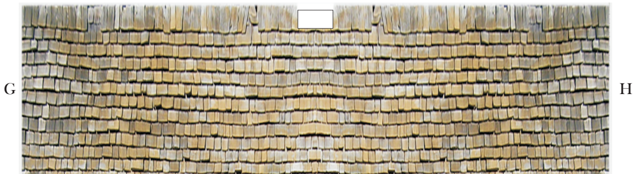
Bottom edge of Front Roof
