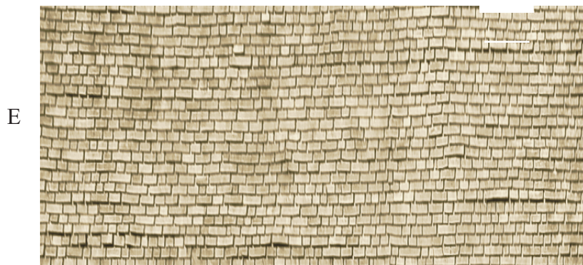
Bottom edge of Front Roof
